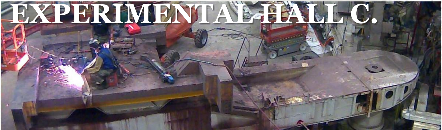
(Removing SOS Floor)
